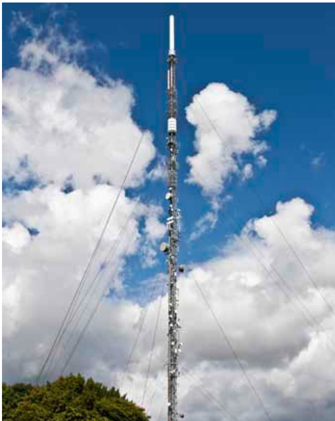
Typical broadcasting antenna.
